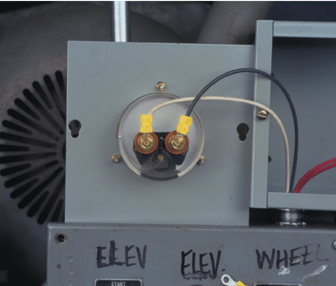
Figure 14. Panel ammeter original wiring
