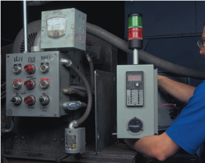
Figure 13. Installation of electrical control panel with AC controller mounted on side
