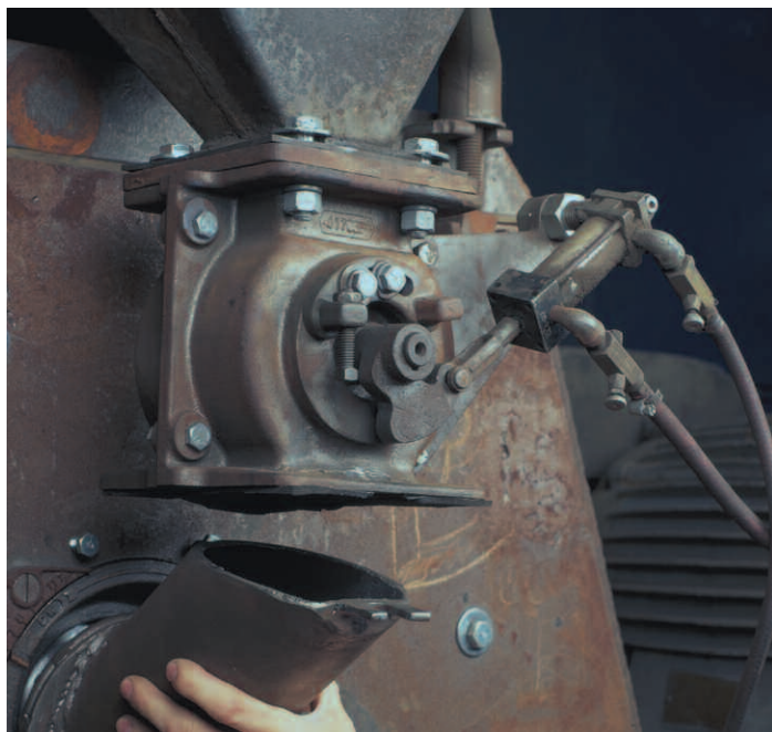
Figure 5. Removing feedspout to wheel
